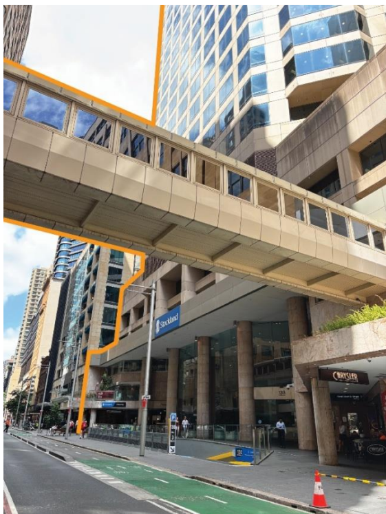
Figure 2: View of the site, in orange outline, from Castlereagh Street looking south
